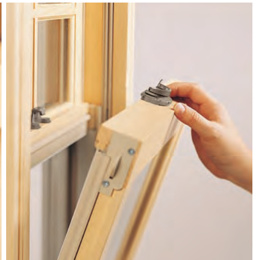
Sash tilting freely into the room.
